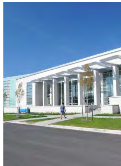
Tech Hall East Entry
