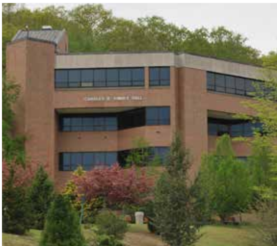
Waterbury Campus Offices & Classrooms: 750 Chase Parkway
