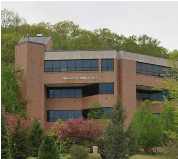
Waterbury Campus Offices & Classrooms: 750 Chase Parkway
